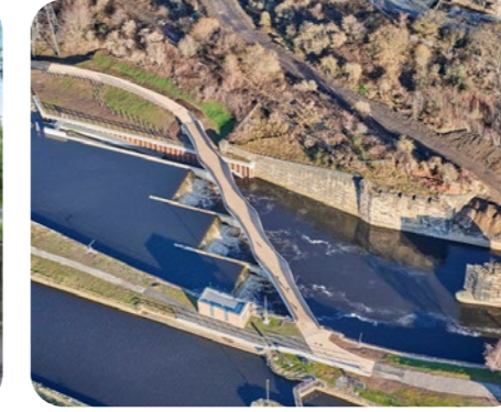
Knostrop Weir, Leeds | Flood Management Provides three new pneumatically moveable weirs that can be lowered to let floodwater discharge quickly downstream.
