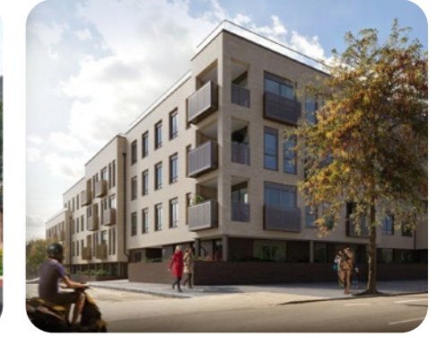
Tallack Road, Waltham Forest, London Large-scale communal Air Source Heat Pump to feed ambient temperature heat network
